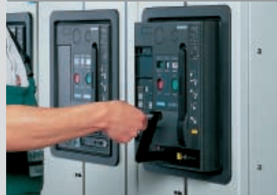
Reliable travel of the circuit breaker while the door is closed
